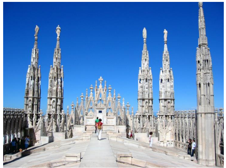
On the roof of Milan’s Duomo (c/o Wikimedia Commons)
